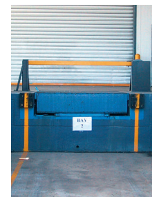
– on external dock
