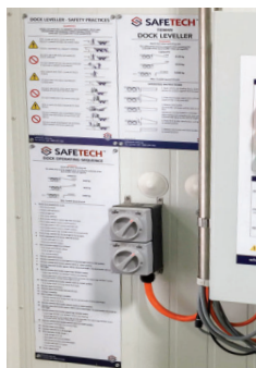
Operational & procedural signage on internal wall
